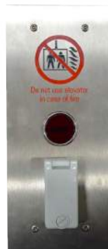
No-entry & Fire-alarm recall key switch (EN81.73)
